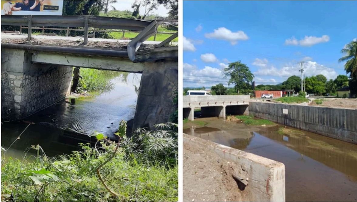
Myton Gully, Jamaica Before and After. Once prone to heavy rainfall and flooding that devastated nearby communities, the upgraded crossing withstood Hurricane Melissa—safeguarding homes, livelihoods, and critical transport routes.
